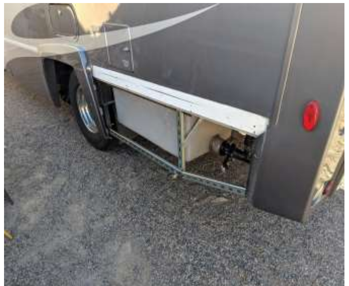
Then I had to weld up a support structure And determine all the mounts and additional hangers.
