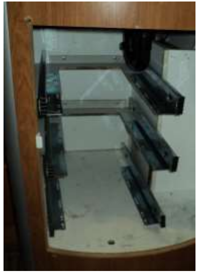
This is the framed in supports for holding the drawers.
